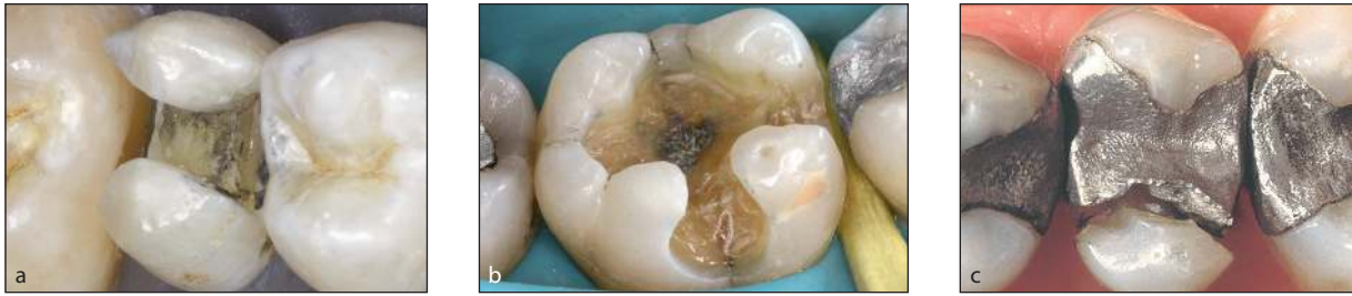
Fig 12-7 (a) The mesio-occlusodistal preparation in the premolar, after removal of a defective restoration, is greater than one-third the intercuspal distance; therefore, the cusps ideally should be protected by reduction and coverage with a restoration, or they should be cross-splinted (see Fig 12-39). (b) The mesio-occlusofacial preparation in the molar leaves facial cusps too thin to resist occlusal loading; they should be reduced and protected with a cuspal-coverage restoration. (c) The lingual cusp of the maxillary premolar, which was not protected or reinforced during restoration, has fractured.
